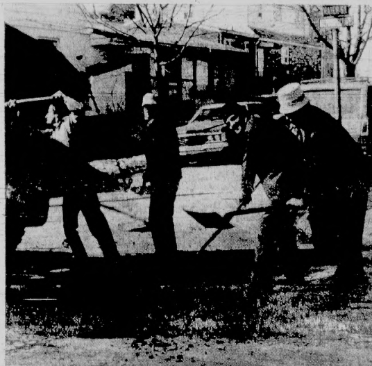
Potholes — The Federal Emergency Unemployment program provided funds to the Department of Public Works and Commissioner Mary Senatore is using the money to fill in the seasonal potholes caused by the recent temperature changes. Above, a Public Works crew applies patches on Mr. Prospect Avenue.
